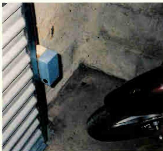
**IR receiver unit mounted at the side of a garage door.**
