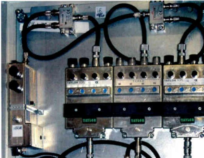
**Figs. 22 and 23:** An arrangement of channel filter/levellers designed to carry five analogue channels and six digital multiplexes. A preamplifier compensates for the combiner and filter losses. The 12dB tap-off unit helps to equalise the channels. The final 6dB combiner is not shown in the photograph.
