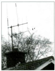
Photo 8: A well-preserved Band I/III aerial for 405-line reception in a good-signal area.
