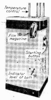
One of the special high-speed processing tanks referred to on the next page.
