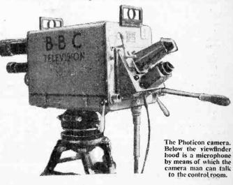
lens mounted parallel to the main or taking lens and focusing a duplicate image of the scene on to a ground glass screen. The two lenses were simultaneously moved by means of a ganged focusing control so that when the image on the ground glass screen was correctly focused, it could be assumed that the other image on the tube target electrode was also in focus.
