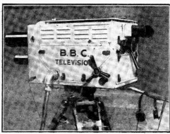
from the unminiaturised image icono- The C.P.S. Emitron camera, with electronic viewfinder. The lens turre scope class to which the E.M.I. Super is controlled from the rear.
