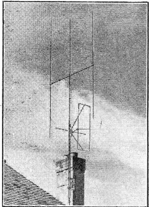
An unusual aerial. This is the J-Beam, combined with a slot aerial for Band III—to be seen on Stand No. 31.
