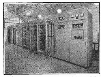
Marconi Vision and Sound Transmitters as used at 1TA London and Winter Hill. The  $7\frac{1}{2}/10$  kW vision transmitter occupies the first seven panels from the right; the  $2\frac{1}{2}$  kW sound transmitter the remainder.
