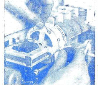
Another splendid illus tration showing the fitting of a New Cord, to the Drum of the to the Drum C. Marconiphone Receiver. 42
