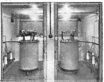
The Baird E.H.T. unit in duplicate as installed in the Marble Arch
