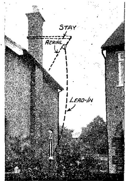
Fig. 6.—Supporting the aerial from a short stay fixed to a chimney.
