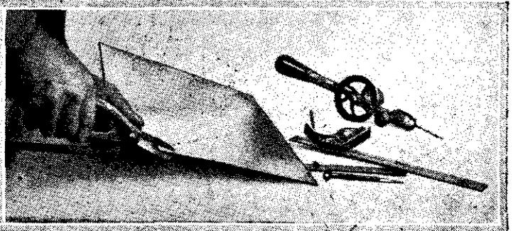
Fig. 8.—How to cut away waste metal without distorting the chassis.
