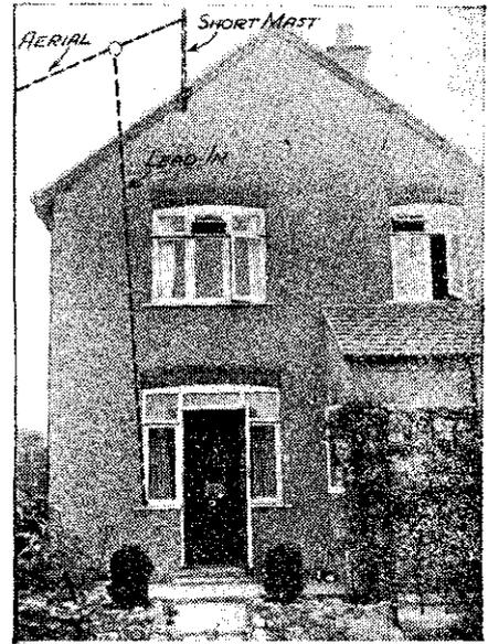
Fig. 2.—Using a short mast for anchoring the house end of aerial.
