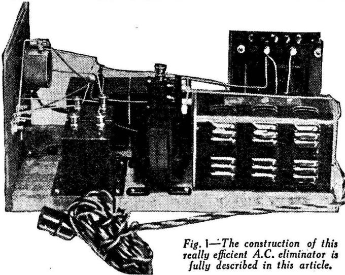
Fig. 1—The construction of this really efficient A.C. eliminator is fully described in this article.
