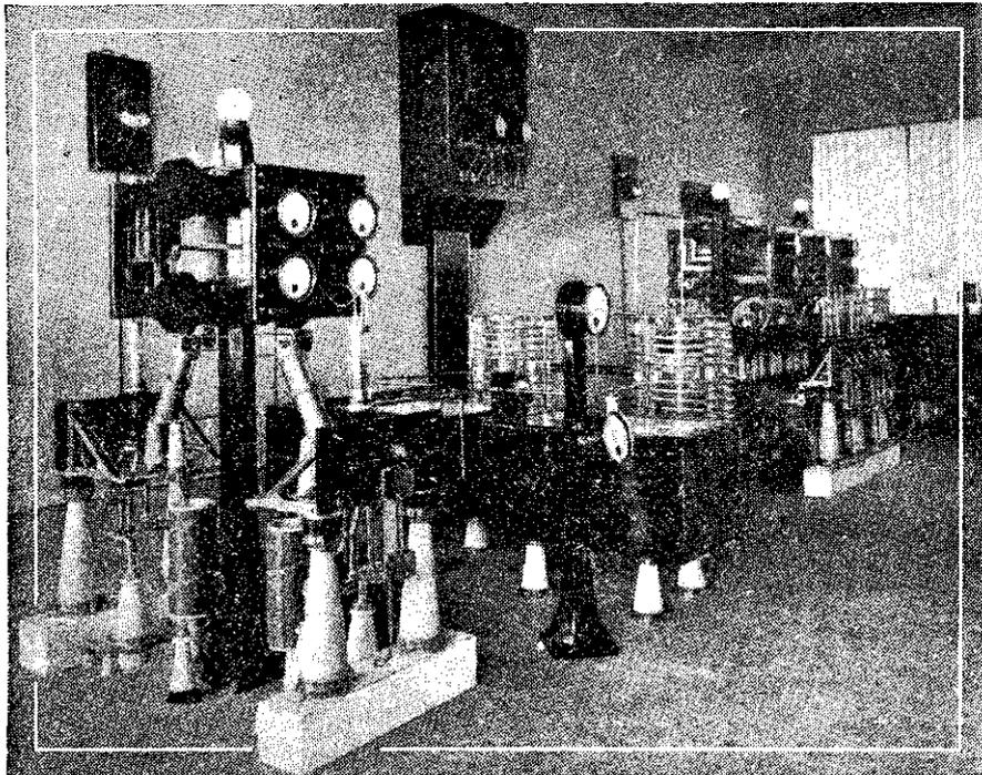
The new radio station is situated in the geographical centre of Europe, some 35 kilometres east of Prague, in the vicinity of the small town of Cesky-Brod. This new high-power broadcasting station is rated at 200 kilowatts (C.C.I.R.), and is the most powerful broadcaster operating in the medium wave broadcast band. The illustration shows: The power amplifier from the front, looking right, at the new Prague broadcasting station.
