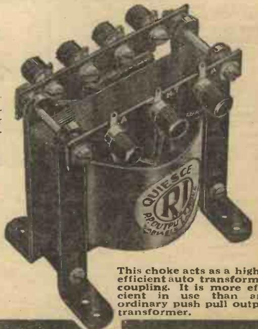
This choke acts as a highly efficient auto transformer coupling. It is more efficient in use than any ordinary push pull output transformer.
