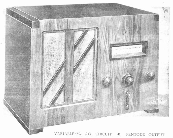
PENTODE DETECTOR \* ENERGISED MOVING COIL SPEAKER
