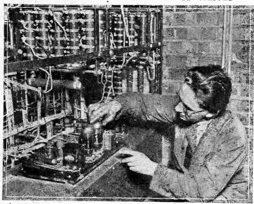
A new system of gearless drive has been introduced to England for the first time in a London building, where sixteen new lifts have just been installed. The interesting feature of this system is that two thermionic valves, such as are used in ordinary wireless sets, smoothly control the stopping and slowing of the lifts, The illustration shows an engineer replacing one of the thermionic valves.
