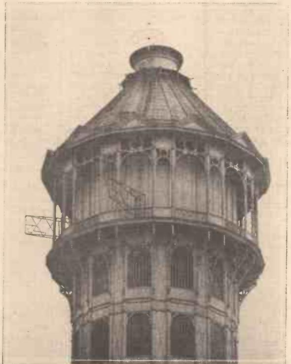
Compare this view of the ultra-short-wave aerial. It may just be seen on the framework projecting from the side of the Crystal Palace Tower. Very little power is required to cover immense ranges on the short waves.
