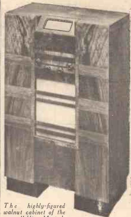
The highly-figured walnut cabinet of the new "His Master's Voice" "Console Superhet Five," Model 444 is of particularly pleasing design. The wave-length scales are set at a convenient angle and the instrument can be operated from an arm-chair. It has a five-valve (including rectifier) superheterodyne chassis, and retails at 17 guineas.
