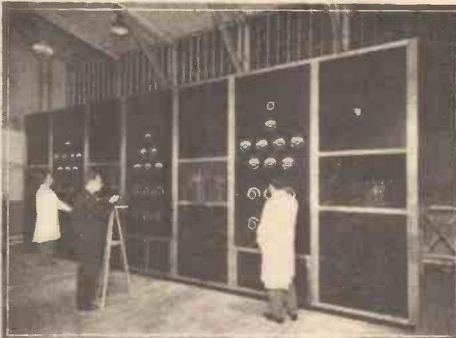
Fig. 4.—The 10-kilowatt ultra-short-wave radio transmitter, which handles the vision signals on a wavelength of 7 metres.
