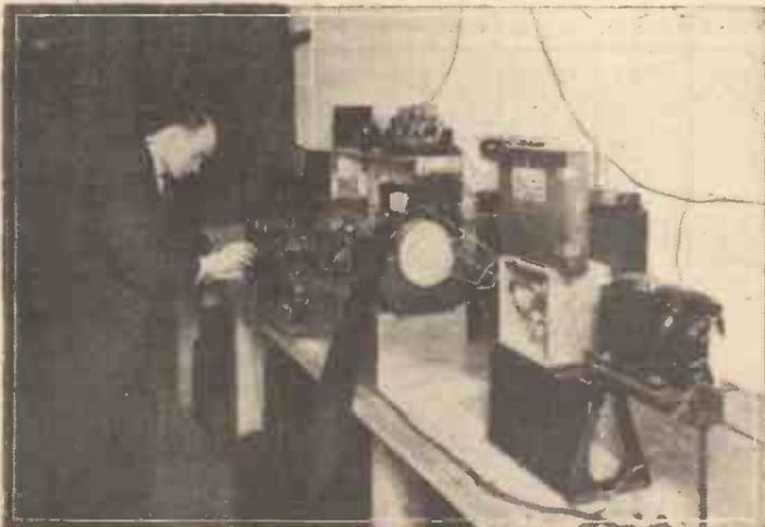
Fig. 5.—Using a cathode-ray tube for recording television images on a film for subsequent projection on to a screen.
