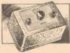
for The experimenter—this is a neat oscillator produced by the makers of the well-known "Avo" instruments, It is known as the "Avo-Oscillator."
