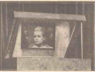
Fig. 2.—A properly-produced 180-line television picture, shown as a masked reflection in a mirror from the end of a cathode-ray tube.
