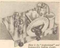
Complete Kit of Parts includes Cossor Valves as follows: Variable-mu H.F. Pentode, H.F. Pentode Detector, and Economy Pentode Output; Super-selective Iron-cored Coils; 8" Moving Coil Speaker; Walnut finished cabinet (providing accommodation for batteries); and all the parts necessary for home assembly.
