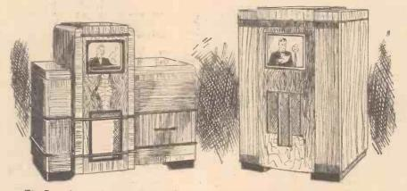
The Pye television receiver on the left incorporates an automatic radiogram. The other Pye model receives the sound and vision programmes only.
