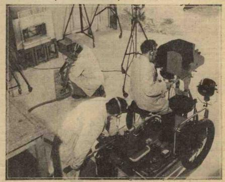
This illustration shows how the television cameras are used to relay both the actual artists and small models which are 'mixed' to provide most realistic effects. The small provides the proscenium and the raising of the curtain before the artists appear. The small model
