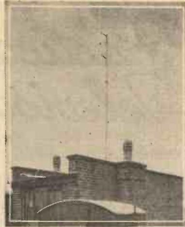
Television aerials on the original Baird Laboratories. Note the solid feeder and the meter inserted in the aerial.
