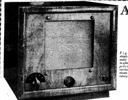
Fig. 1.—A simple automatic receiver in which station selection is carried out by means of a rotary switch.
