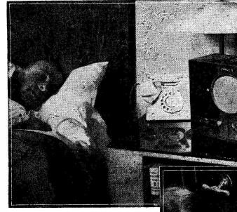
These illustrations show how a shopkeeper protects his safe by placing a Philcophone underneath it where it cannot be seen. Should anyone approach the safe, the slightest noise will be intensified in the master unit, in his bedroom upstairs, sufficiently to awaken him.
