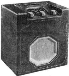
This is Invicta New Junior Portable. It employs a 4-valve circuit and has a P.M. speaker. The size is 12½in. by 12in. by 8¾in., and the weight 20lbs. Total H.T. consumption is approximately 10 mA, and the output 200 mW.
