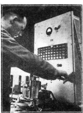
Here is a factory tester which does all circuit testing without dismantling any parts or leads. It is in the G.E.C. factories.
