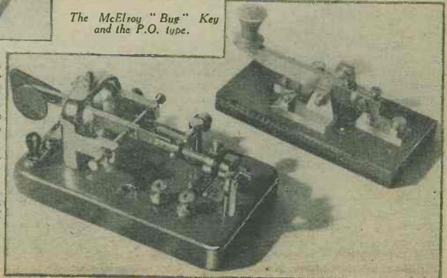
McElroy "Bug" Key, which operates on a semi-automatic principle. Whilst this type of key is widely used in America, and is, of course, directly connected with the record breaking achievements of McElroy, the American Morse specialist, Messrs. Webb point out, that the key is now unobtainable in this country, and has been submitted solely out of interest and to form a comparison with those of the more standard types.
