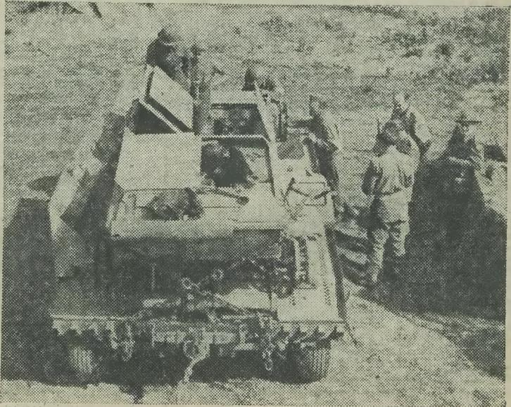
The first German radio-controlled tank captured at the Anzio Bridgehead. It is 12ft. long and 6ft. wide, and carries a high explosive charge of about 800lb.
