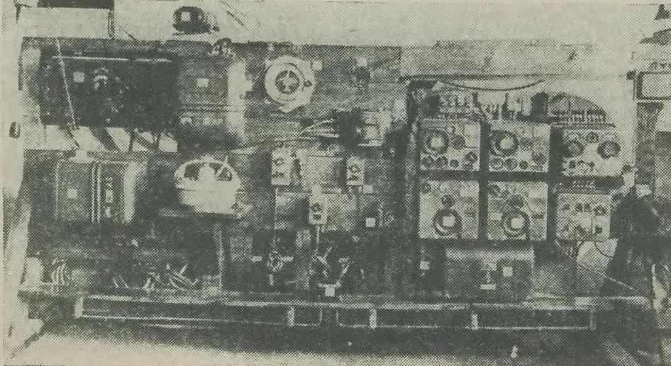
receiver fine-tuning prevented the pilots from getting the best out of this apparatus, whilst its replacement by the FuG 16 was much overdue. The continued use of the FuG 7a for fighter R/T was thought to indicate the Germans' reluctance for re-equipment during the war as well as their preoccupation with bomber radio devices, to the detriment of defensive aircraft.
