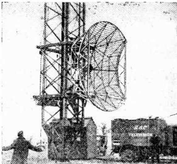
A close-up of the G.E.C. paraboloid aerial and mobile television laboratory used in recent television link field trials.
