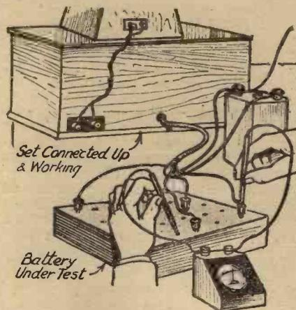
Test the H.T. battery when the set is working.
