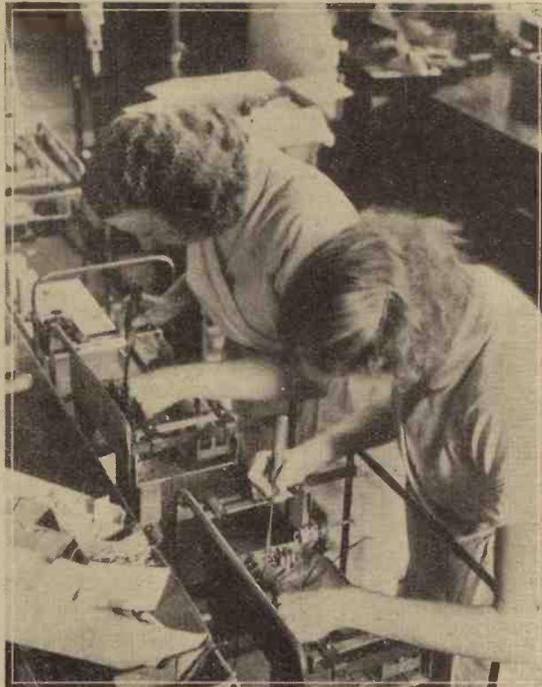
The start of an assembly line. Note how the chassis are safeguarded by the protecting steel cradles.
