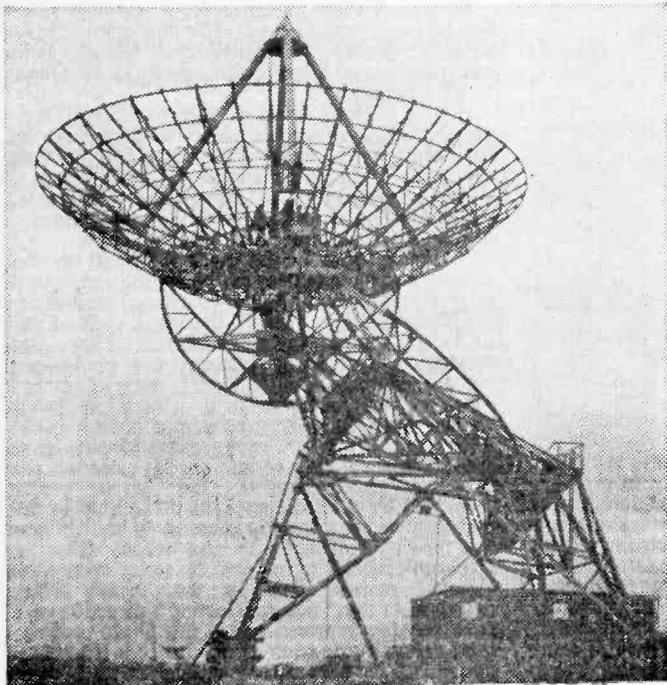
*This illustration shows the central, fixed aerial of the new radio telescope at Cambridge. Underneath this aerial is its control building and just visible above the skyline is the movable aerial.*
