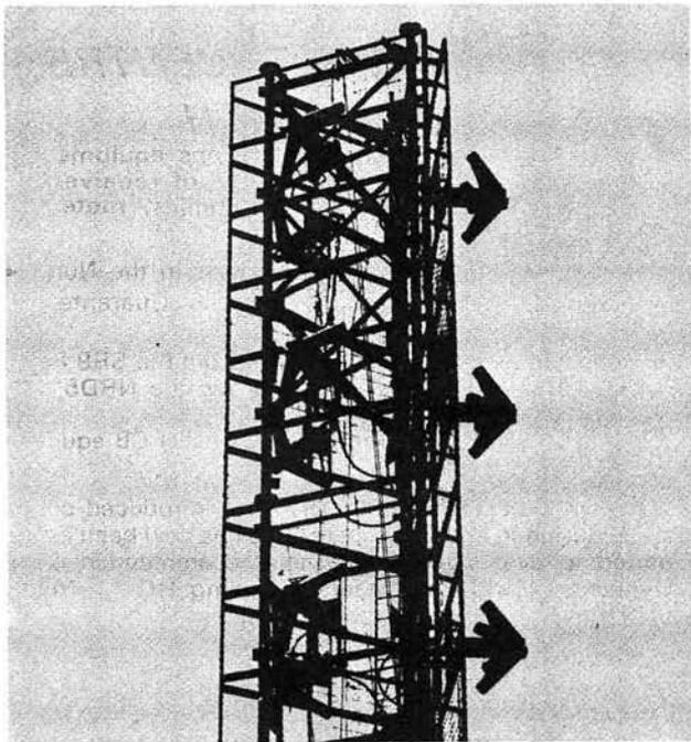
◀ A close-up of part of the crossed-dipole array at one of the BBC's v.h.f. relay transmitters
