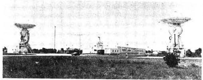
STDN ground station provides communications with the Orbiter during launch and landing (NASA)
