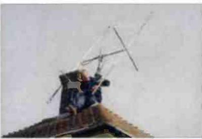
Fig. 2: The reflector assembly being fixed to the end of the boom.
