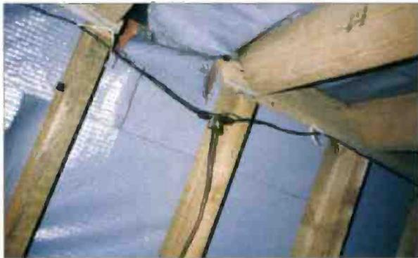
Fig. 3: Photo showing the centre feeder connection of the h.f. antenna. The conductor is supported to the timbers by a cord, while the helixes are wound on roof timbers insulated by a plastic membrane (but large diameter plastic piping could be used as an alternative).
