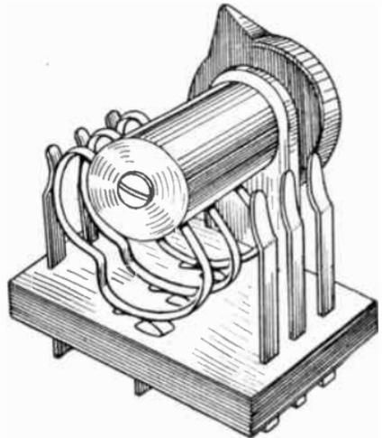
FIG. 382.—Another form of low-capacity Switch.
