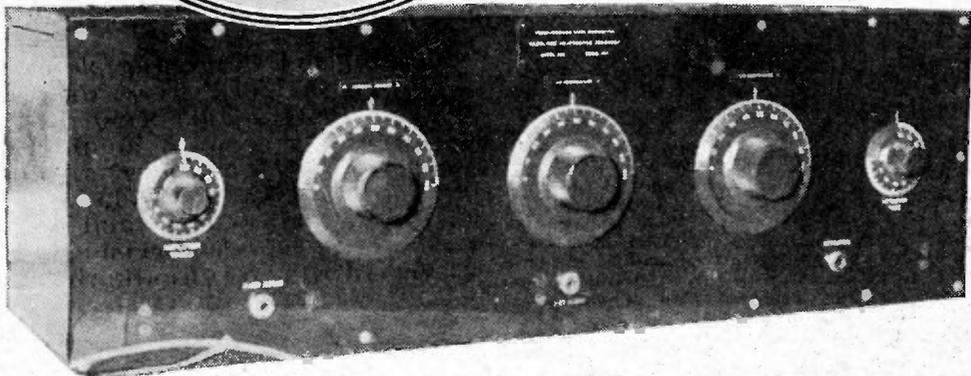
A typical example of American design—the exterior view of a Neutrodyne Receiver.
