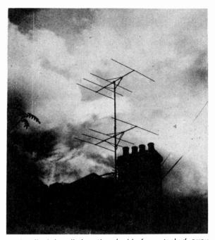
In the final installation the double-four stacked array shown here was used for the ch. F2 vision. This was erected on an 18ft. mast and used cut down versions of ch. B2 arrays. The separate sound aerial is mounted on another chimney.
