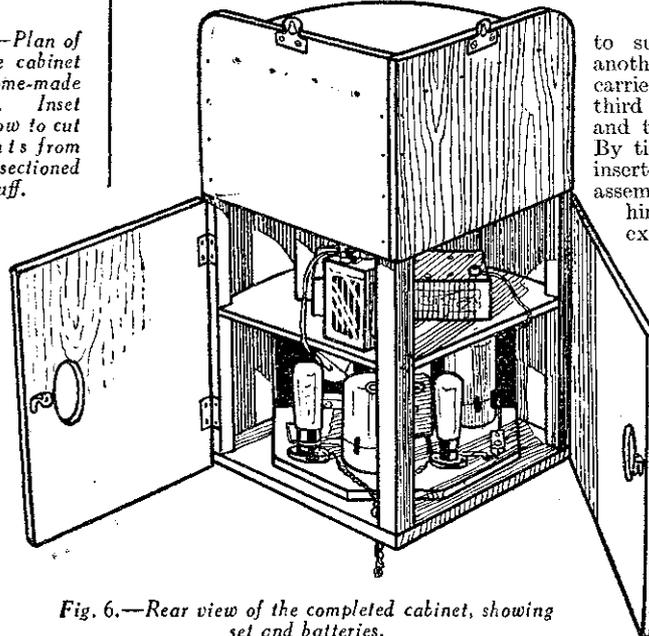
Fig. 6.—Rear view of the completed cabinet, showing set and batteries.
