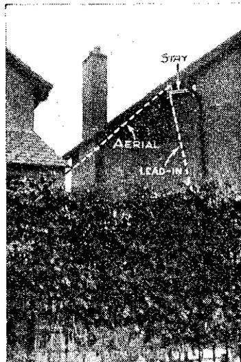
Fig. 3.—A stay can be used for keeping the lead-in away from the house wall.
