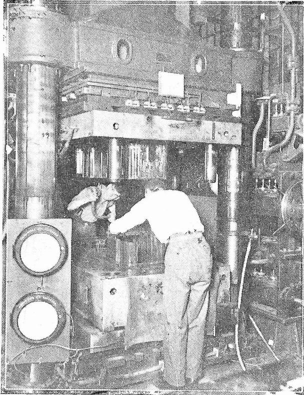
How bakelite is moulded at the Ekco Factory. (See the paragraph on this page.) This press produces two Model 74 Cabinets at one stroke.
