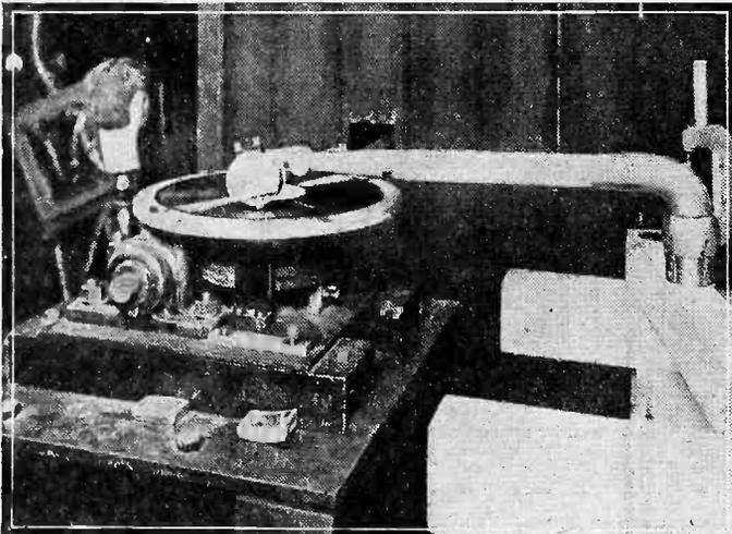
Fig. 2.—A dummy's head acting as the subject for making a test phonovision record, this latter process being visible in the foreground.
