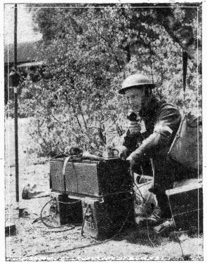
A modern portable field radio transmitter and receiver. Note the aerial-earth arrangement and battery supplies.
