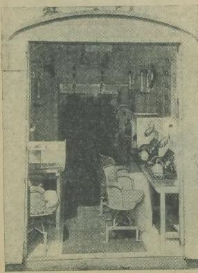
View of receiving vehicle. Reading right to left are two perforating positions, one undulator with receiver and bridge above, one Wheatstone transmitter, then second undulator with second receiver above and two take reading positions. Desk on front left is the superintendent's desk.
