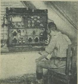
This equipment, forming a mobile transmitting station in Ceylon, is subjected to high temperatures and humidity.
