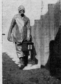
With a risk, in an air raid, of failure of the with a risk, in an air raia, of fature of the electricity supply, battery portables have distinct advantages for A.R.P. work. This portable, working 10ft. below ground level in the Ekco radio shelter at Southend-on-Sea, gave results identical with those obtained in normal conditions on the surface.
