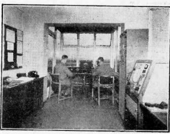
The Marconi AD.200 VHF DF installation in the control tower at the de Havilland airfield, Hatfield. On the right can be seen the master control console and the twin receivers, and in the centre of the aircraft control officers' desk is a remote bearing indicator and twin loudspeaker.—See page 8.
