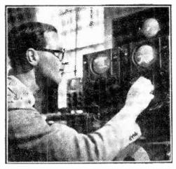
In one of the laboratories at the Shrivenham Military College, Berks, are three radar screens. two of them move patterns transmitted by instruments at the other end of the laboratory. The top screen is the face of a "radar clock" whose hands tick off the minutes and seconds, the hands being strips of green light and the works a circuit of radio ralves
