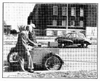
Demonstrating the radar speedmeter on the Cromwell Road extension at Hammersmith. In this picture are the R.A.C.'s chief engineer Mr. Maurice Hudlass of Southport, Lancs., and Patrolman Arthur Isherwood of Tooting, London, They are seen checking a car passing the radar speedmeter.
