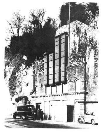
The entrance to the BBC's wartime Bristol HQ showing ventilation intake and outlets. Adjoining these on the right is the antenna mast for reception
