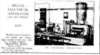
The receiver was tuned by a two-slider inductance and a selection of different detectors, including the popular Perikon type. This photograph was widely known as it appeared on the cover of the Gamages Directory of Experimental Wireless Stations in the UK.
