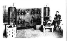
Mr. W. T. Ditcham, a Marconi engineer and the world's first broadcaster at the 6kW transmitter used in his original experiments
