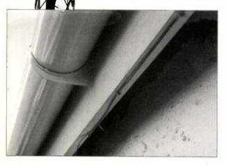
Fig. 2: The wire under the eaves would not be seen at all if it were fitted behind the facia or behind the soffit board.
