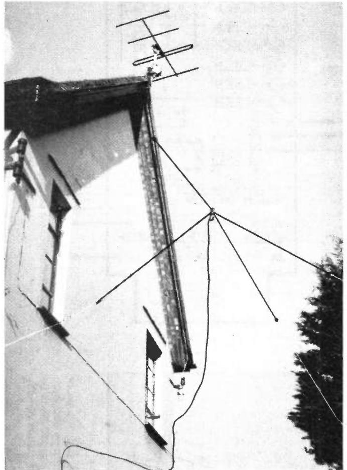
Figure 1. Arrangement of 10 metre crossed dipole antenna, showing coiled up stub, matching section and feeder. 2 metre Yagi with directional control on pitch of roof.
