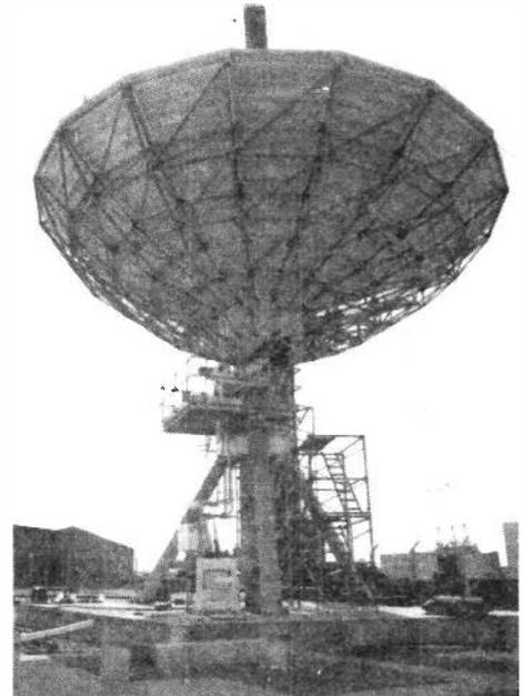
The new 13 metre satellite earth station antenna, known as System 2, under construction by Marconi Communication Systems Ltd for Mercury Communications Ltd at the Isle of Dogs in London
