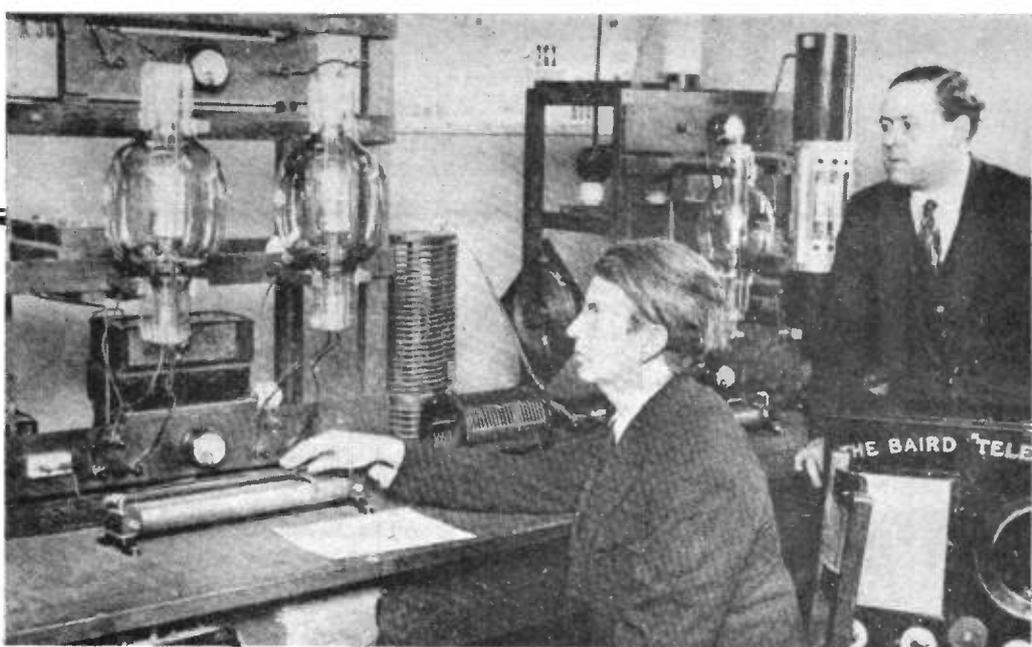
The amateur transmitter used for the first transatlantic television transmission in 1928. J L Baird (sitting) and Ben Clapp G2KZ
